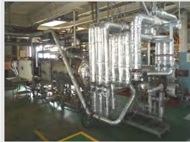
100kg/h single burner test furnace - Concept verification
