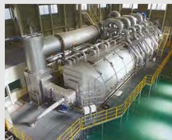
4t/h single burner test furnace - Burner performance confirmation
